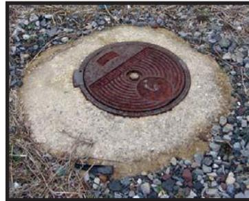
Groundwater monitoring wells both on- and off-site are used to identify potential impacts from MGP by-products in groundwater.
