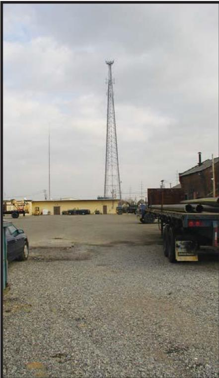
A combination of asphalt, an office building and crushed rock and clean soil creates a protective covering over the former MGP property.
